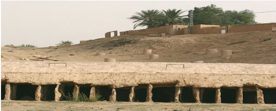
Figure 5. Tissebath and ventilation shafts.
