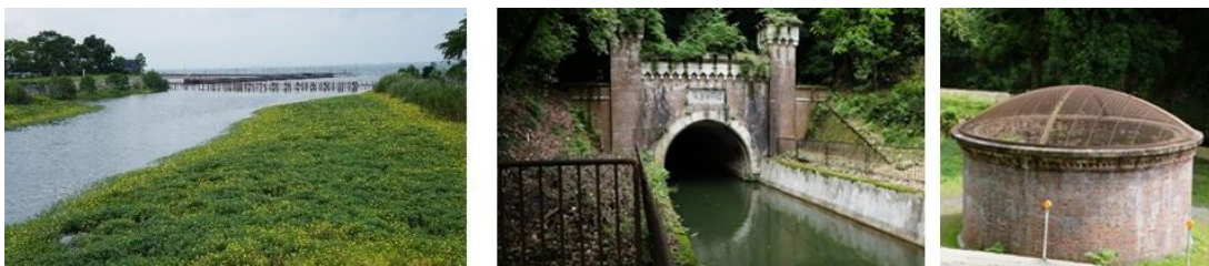
Figure 3. The beginning of Lake Biwa Canal, the entrance to the First tunnel and the head of the first tunnel shaft (by author).
