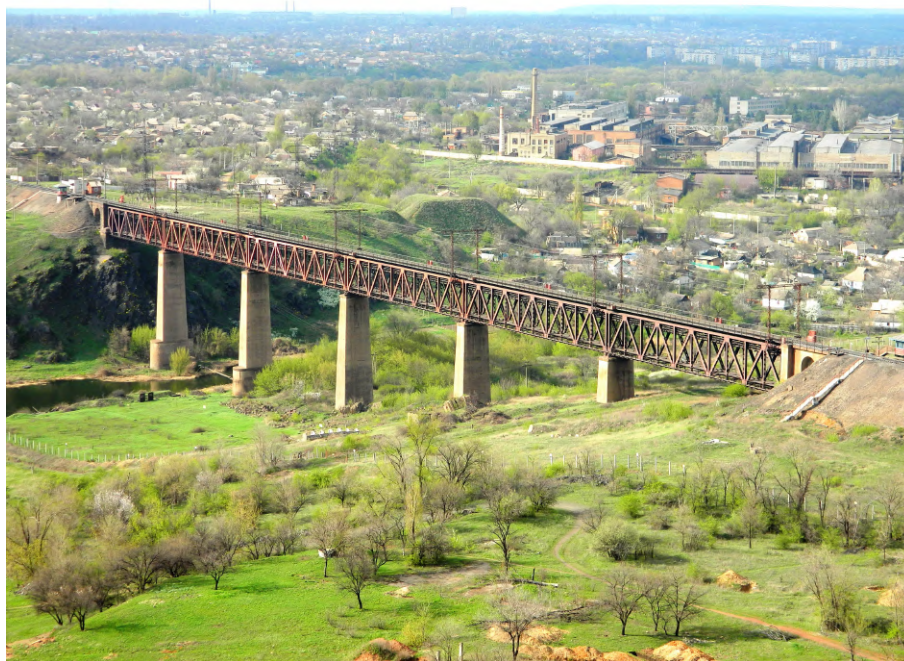
Figure 3. Panorama of Beleliubskiy bridge and the city from the Burshchytskyi dump (photographed by V. Kazakov).
