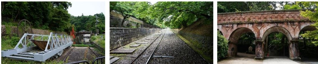
Figure 4. Keage Incline and Nanzenji Suirokaku aqueduct (by author).
