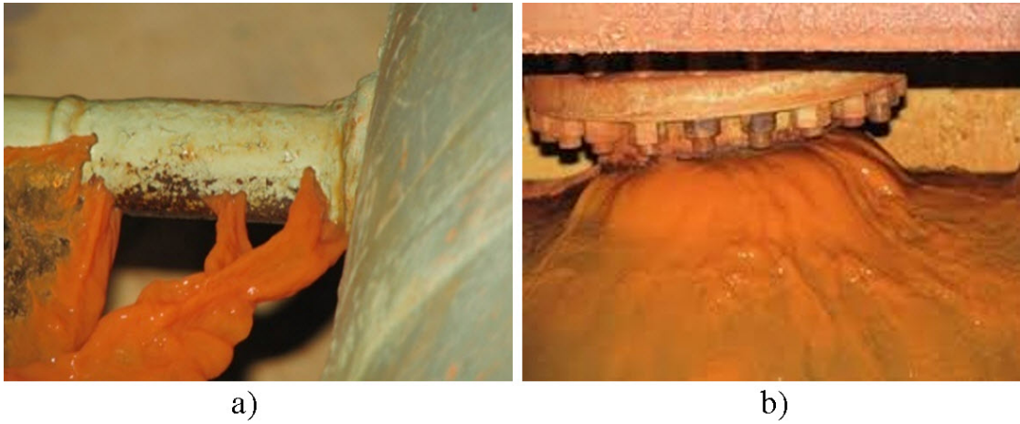
Figure 1: Photos of the accident with the spill of radioactive decontamination solution at the Ignalina NPP (Lithuania, 2010): view of the broken pipeline (a), general view of the spill part (b) [34].
