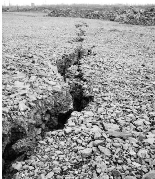
Fig. 1. Scheme of forming cracks on the northern side of the Open Pit No. 1 of the Mining and Processing Plant “Novokryvorizkyi GOK” (formation of terraces)
