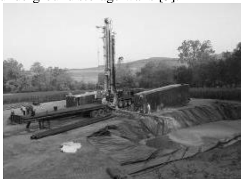
Fig. 1. General view of the storage of waste [6]
